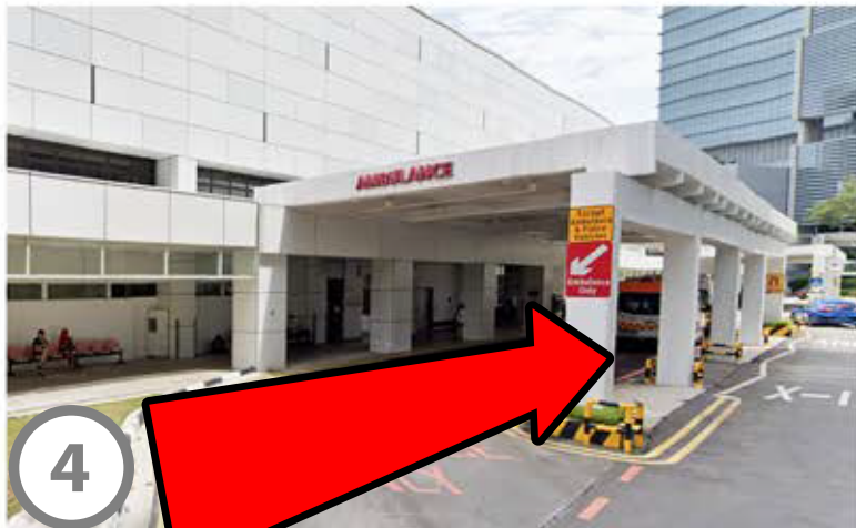
Follow the hospital path, walk pass the Emergency department and ambulance bay .
