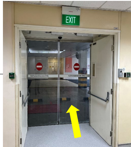
Exit to Ambulance Parking Bay
