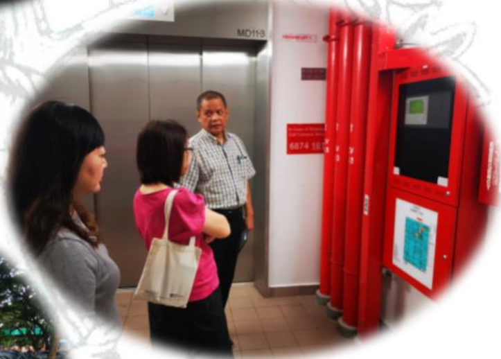
Familiarization of fire emergency warning devices such as Fire Alarm Panel and bell and procedure if they are activated for MD11 B1
